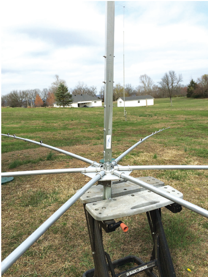
Figure 20 — Spreader plate with the center post and spreaders installed. Note studs sticking out for future wire attachment
