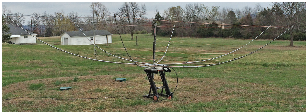
Figure 22 — Support cords pulled into place.
